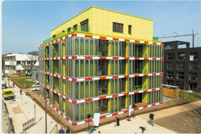
FIGURE 13.17 The algae-powered Bio Intelligent Quotient House in Hamburg, Germany
